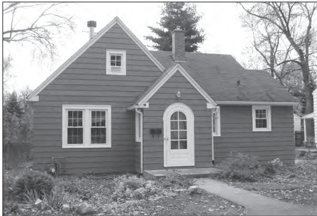
Sears Catalog prefabricated home at 4021 Winnemac Avenue built in 1939. (Photo taken in 2010.)
