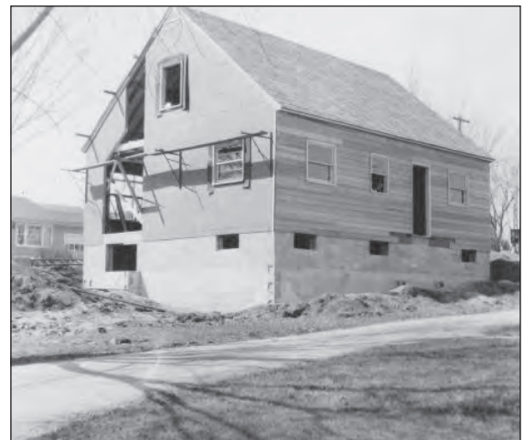
The Jackson’s house at 461 Westmorland Boulevard under construction in 1951.
