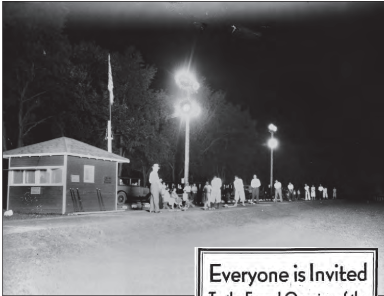
The Speedway Driving Range billed itself as the first illuminated driving field “in the middle west.” The ad proclaimed, “The new General Electric Lighting System gives perfect illumination all over the field. You are able to follow your ball even better than in daytime.” (WHi 20301)
