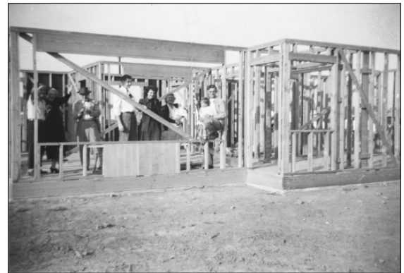
The Martinelli’s house at 4318 Tokay Boulevard under construction in 1949.
