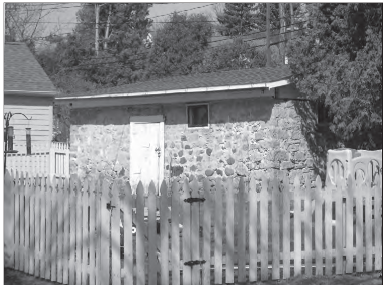
A “mystery” building at 3822 Paunack Avenue was most likely built to serve as a farm shed for Charles Baker’s Sunnyside Farm.
