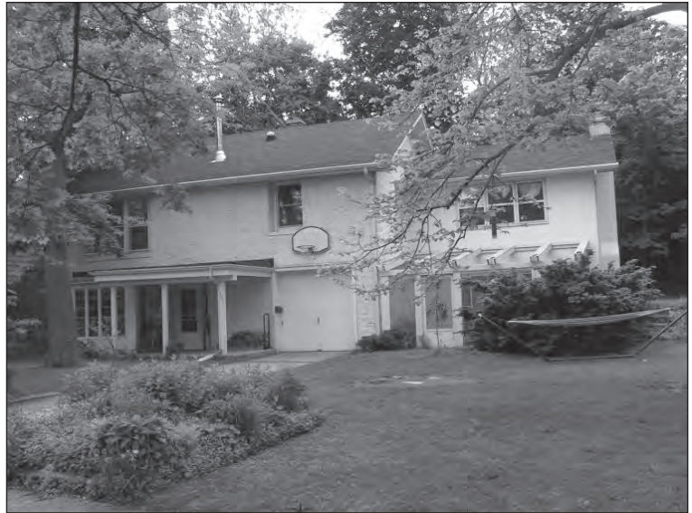
The oldest building in Westmorland, at 4010 Paunack Avenue, was built in about 1860 to serve as a stable for Charles Baker’s Sunnyside Farm.
